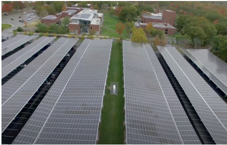
Bristol Community College's Solar Array
